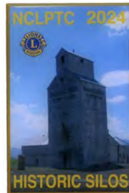
FG 1201 24 Bob Walker (SC) Silo # 7
